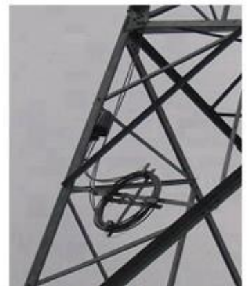
Picture 17: Installation of Downlead Clamp, Cable Tray and Joint Box.
